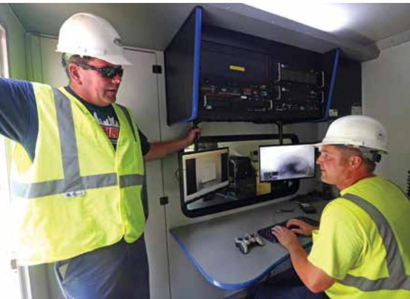
Owner Chuck Lang (left) speaks with camera technician Kevin Lyons about a lateral assessment job in the control room of the inspection van.
