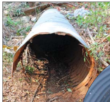
This culvert beneath a road had deteriorated badly.
