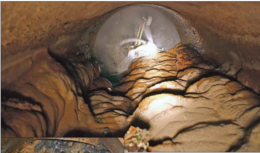
A tool is shown cutting through some of the toughest lime deposits. Bottom photo: The chain scraper is sent through the manhole to clean the invert and the beginning of the adjoining line.
