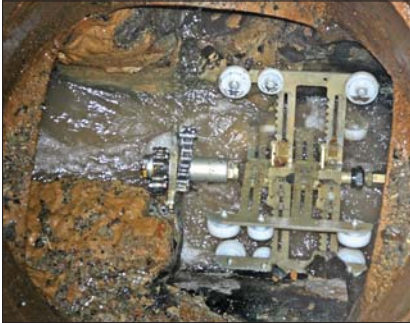
A tool is shown cutting through some of the toughest lime deposits. Bottom photo: The chain scraper is sent through the manhole to clean the invert and the beginning of the adjoining line.
