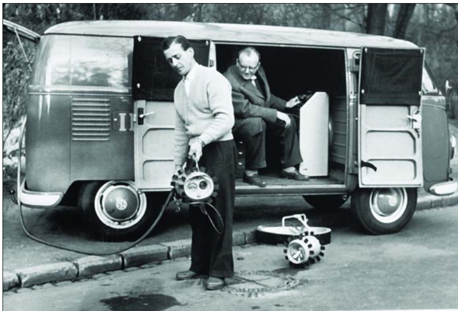
An example of what the first camera inspection trucks looked like, circa 1958.
