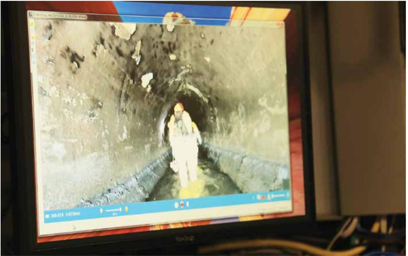
*Manned entry for sounding and core sample collection required a significant health and safety work plan*
