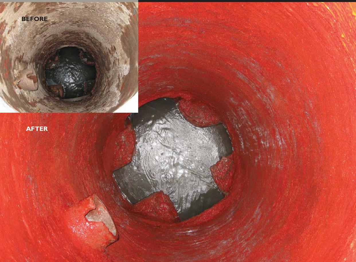
A manhole is shown before and after lining with the epoxy coating system. (Photos courtesy Wastewater Collection Division, Miami-Dade Water and Sewer Department)
