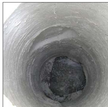
**The concrete polymer paste restores manholes by filling voids. This manhole is ready for coating.**
