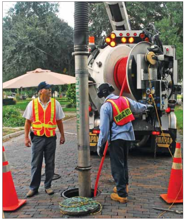
Above, the Quick Television crew from the city's Preventive Maintenance Section uses a pole camera to inspect sewers. Operating the camera is wastewater technician DiMario McKenzie. Right, wastewater technician John Martin cleans a line as wastewater collections system maintenance division manager Lane Longley observes.
