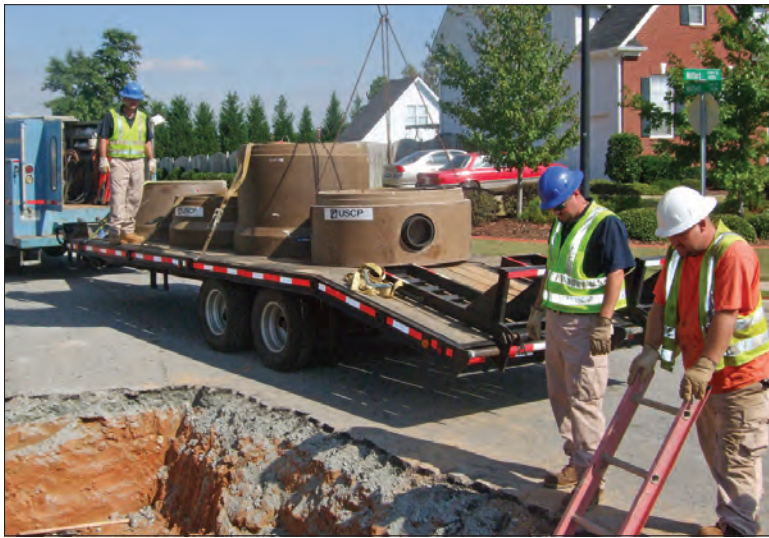
Gwinnett County workers prepare to install the sections of a composite manhole.
